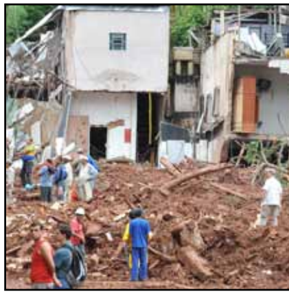
Figure 5: Landslide damage in Nova Friburgo
